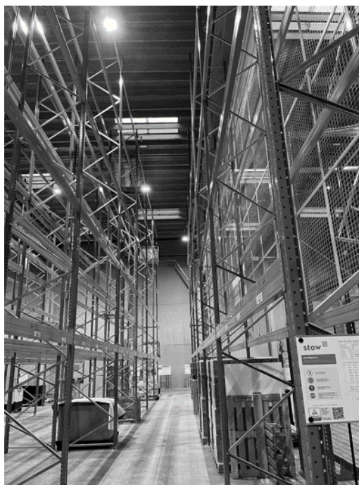
Figure 34: Picture of the metal racks in the pallet warehouse.
